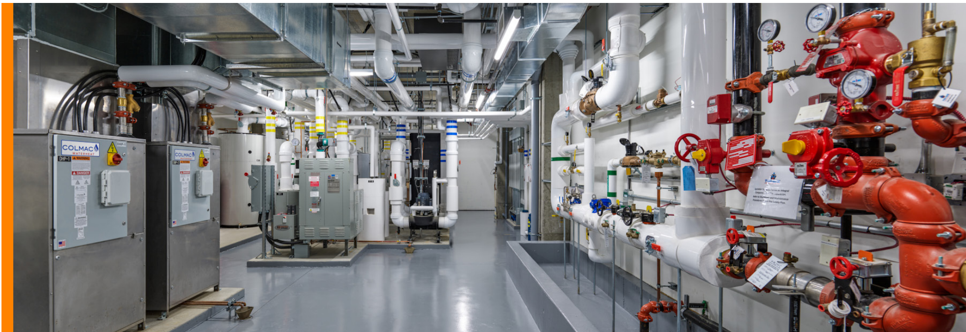
Mechanical room on the ground floor. (Credit: Andrew Latreille.)
