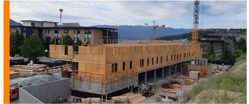
Construction of the wood-framed structure over the ground floor. (Credit: Sawchuk Developments Co. Ltd.)
