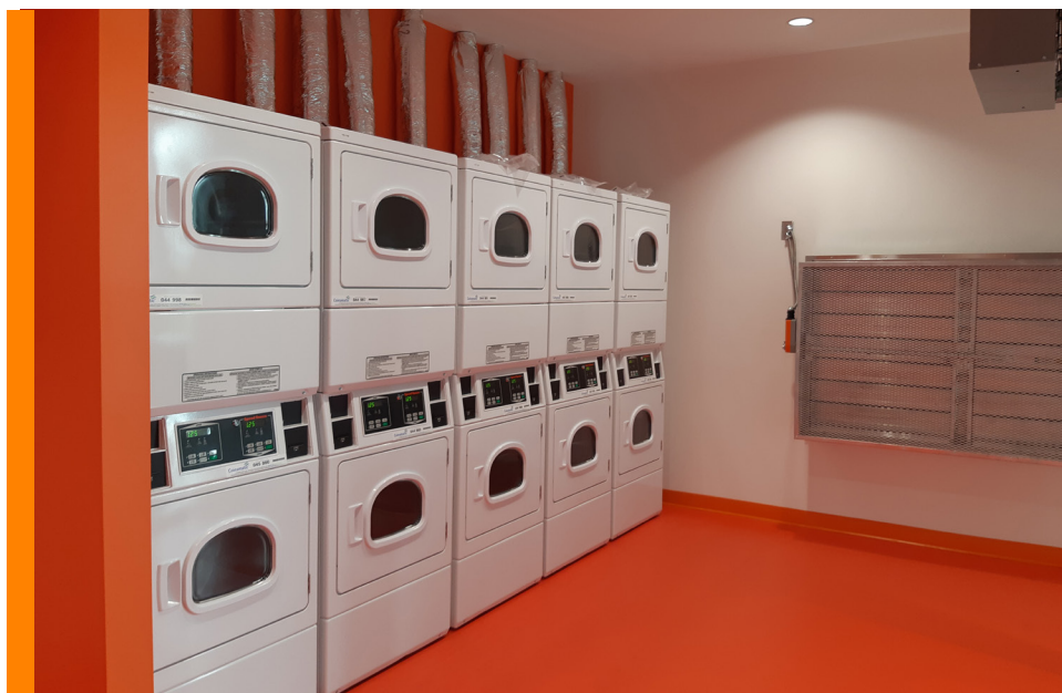
Conventional dryers and make-up air damper (Credit: Sawchuk Developments Co. Ltd.)
