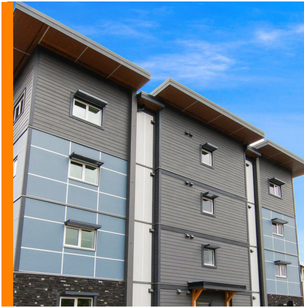
Carrington View Building A (Credit: Skyline Living)
