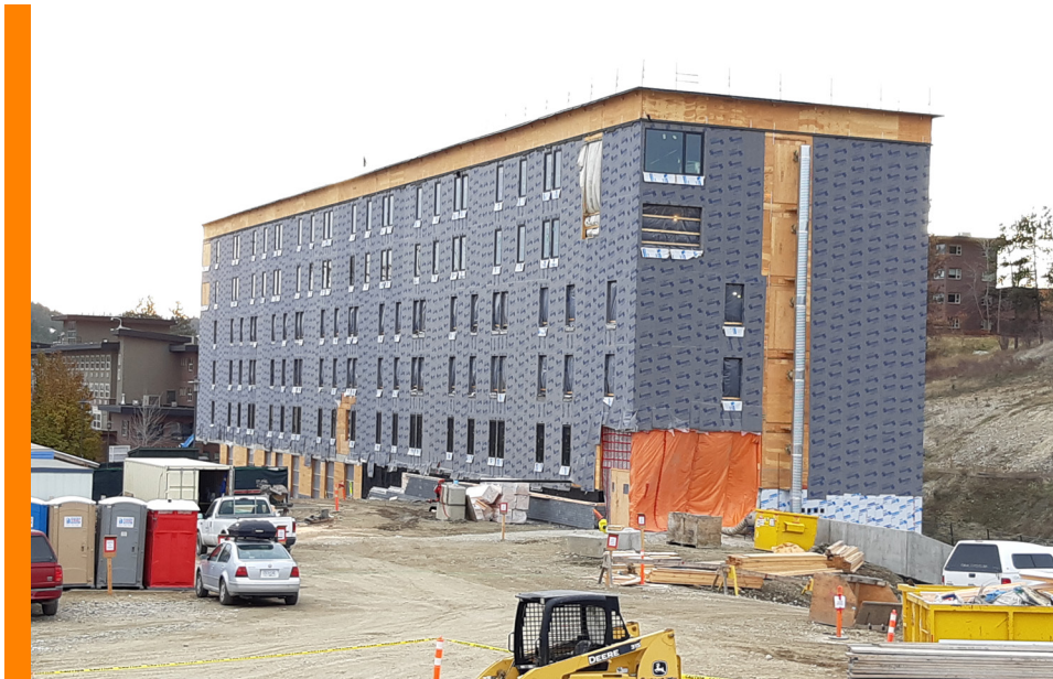
Installation of the air barrier. (Credit: Sawchuk Developments Co. Ltd.)
