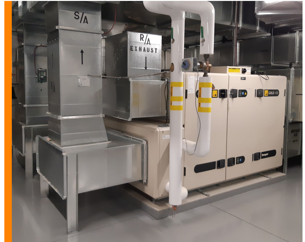
Swegon ERV (Credit: Sawchuk Developments Co. Ltd.)
