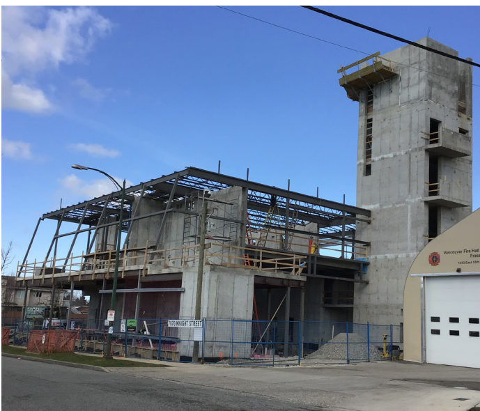
Fire Hall No. 17 construction site (Credit: HCMA)
