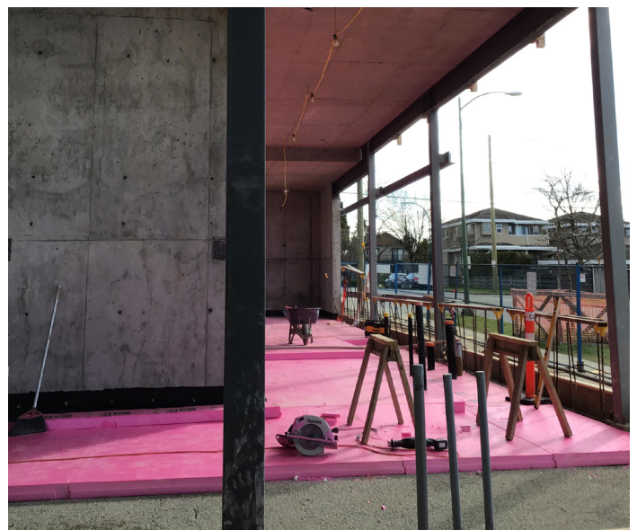
Slab on grade insulation installation (Credit: HCMA)
