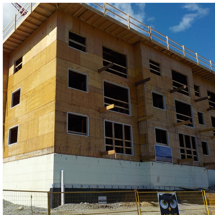
Orion's envelope is constructed with a highly insulated 2x6 stud wall on the inside and an exterior insulation and finish system (EIFS). It also has a liquid-applied vapour barrier (Credit: Vidorra Developments Ltd.).
