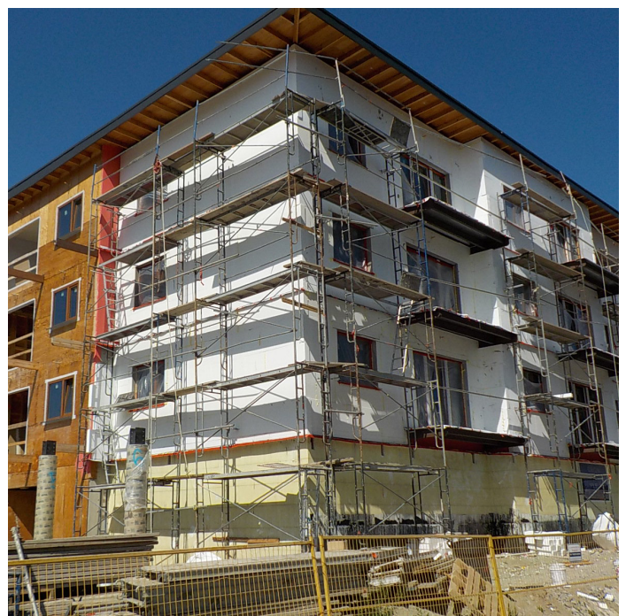
Orion's envelope is constructed with a highly insulated 2x6 stud wall on the inside and an exterior insulation and finish system (EIFS). It also has a liquid-applied vapour barrier (Credit: Vidorra Developments Ltd.).
