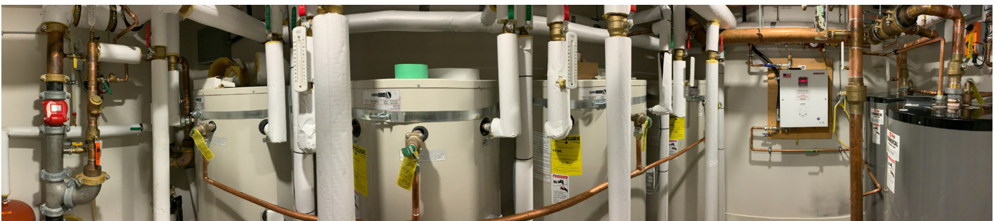
Top left: Eight Sanden CO 2 air-to-water heat pumps are used as a primary source to heat the DHW for the building. Top right: Wood is used as the main material for the structure and envelope to reduce the building's embodied carbon. Bottom: DHW system uses a 27kW supplementary electric boiler for back-up. DHW system design incorporates highly insulated piping and an efficient monitoring and control system to prevent unintended heat losses. (Credit: Vidorra Developments Ltd.)
